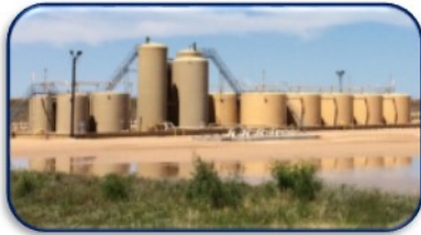
LMS Water Treatment Plant
