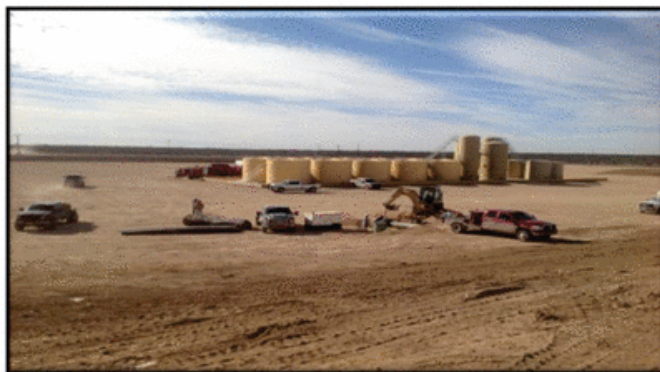
Water Recycle Facility (Under Construction)
